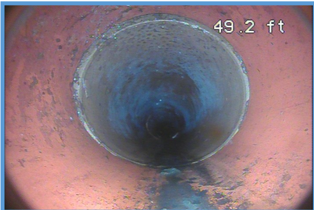
Clean, well sloped clay pipe. Note the obstruction free joint
