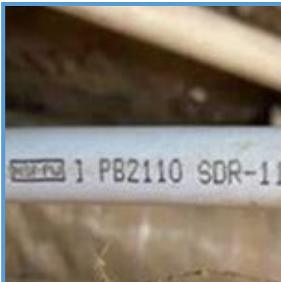
Grey Polybutylene pipe with PB2110 label
