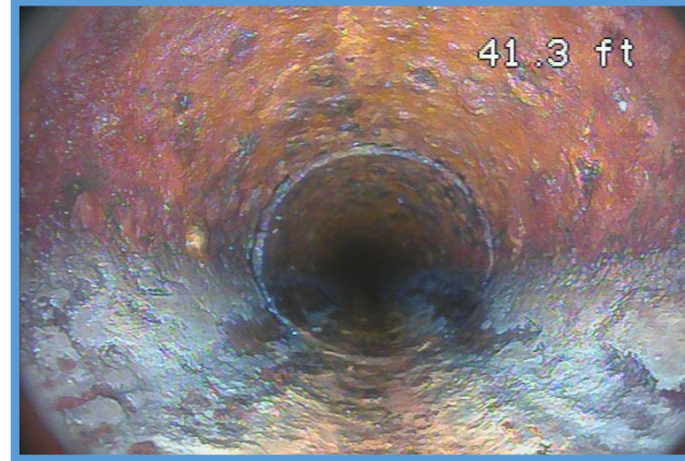
Clay pipe with root mass partially blocking the pipe
