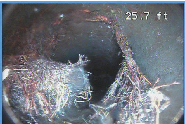
Clay pipe with root mass partially blocking the pipe
